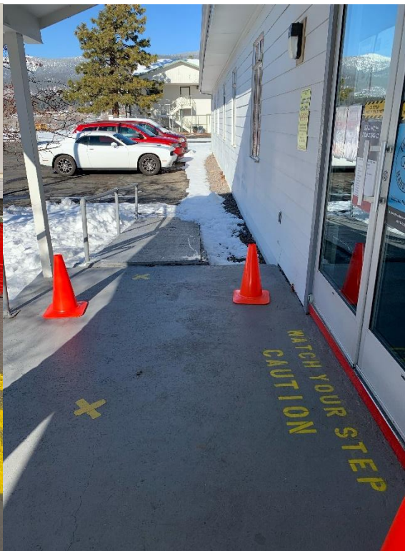
7 Main Entrance Landing
